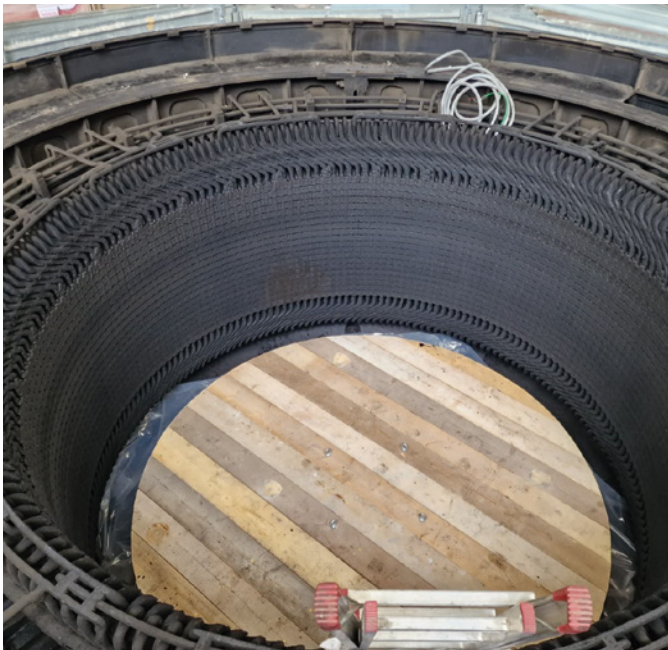
ABB spa, Electric generator maintenance
