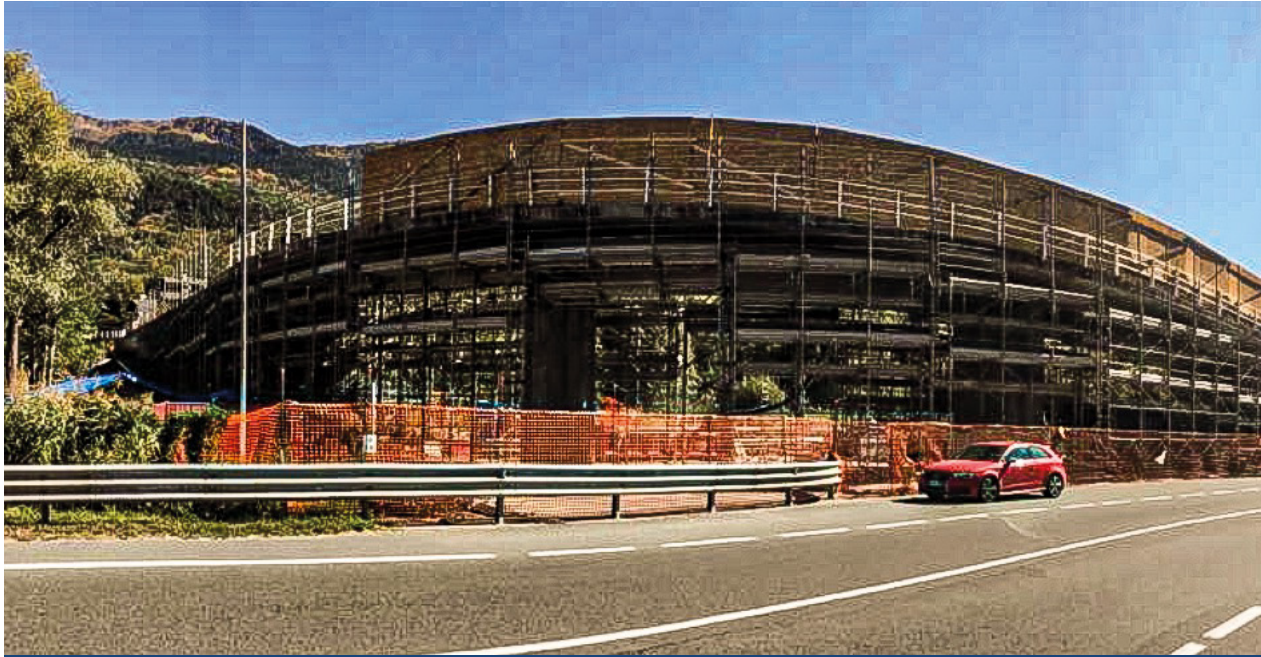
Railway Bridge, S.S. 54 Sarre (AO)
