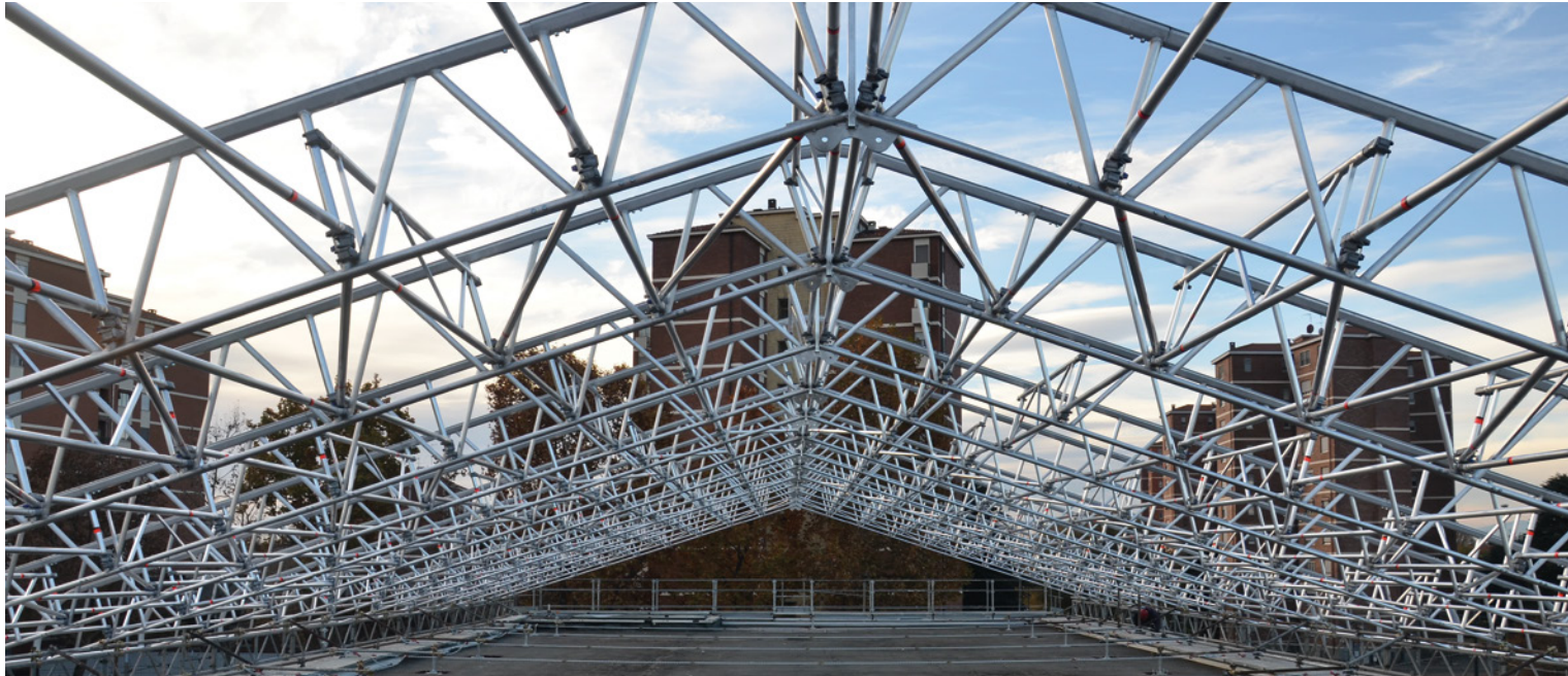
Temporary Covering in Via Crispi, Varese
