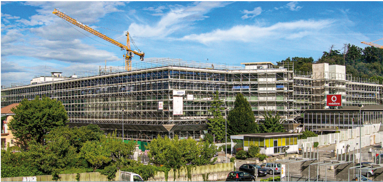
Former Olivetti Headquarters, New Vodafone Offices, Ivrea (TO)
