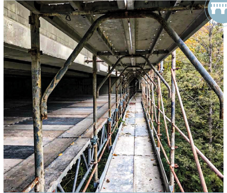
Bumaz Viaduct, S.S. 27 Km 11+618 (AO)
