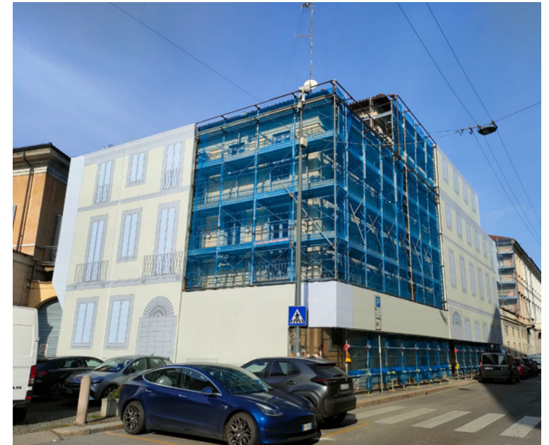
Advertising Structure in Via Manin, Milano
